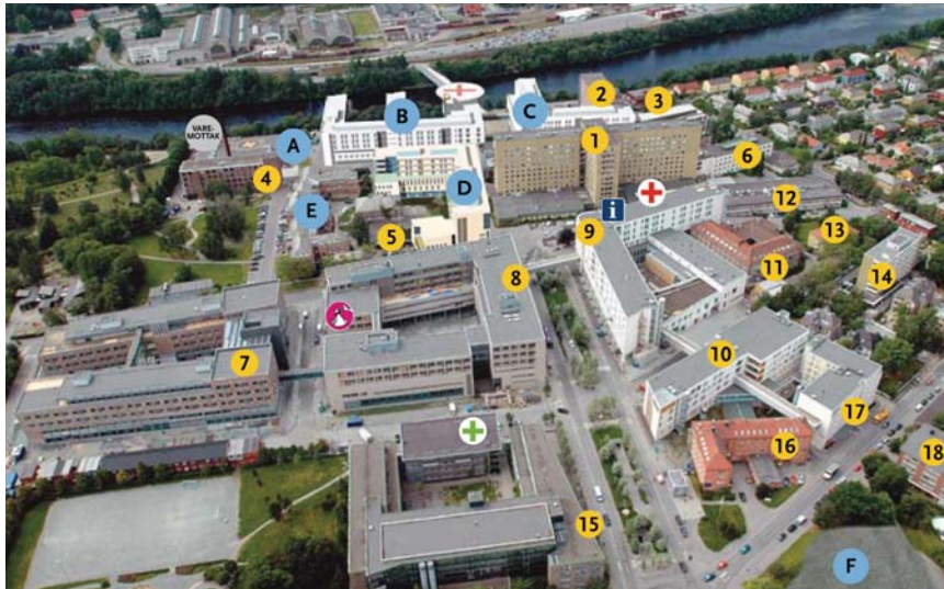
Aerial Site View
