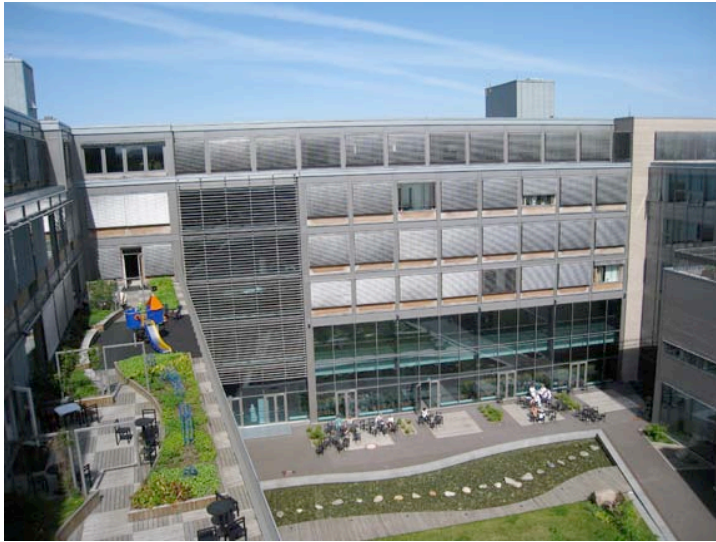
Figure 8.0: Central Courtyard at St. Olav's Women and Children's Centre, Trondheim Norway. This hospital maximizes places to be, and places to see outside even in an urban setting.
